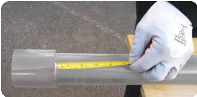
8. Using the mark previously made, check that the pipe has been fully inserted.
